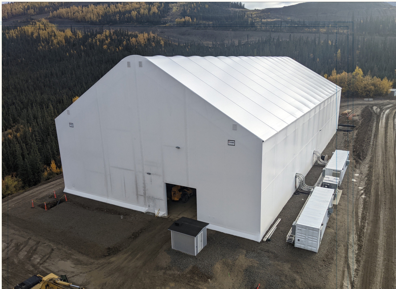
Victoria Gold's Water Treatment Plant at the Eagle Gold Mine, constructed in 2022.
