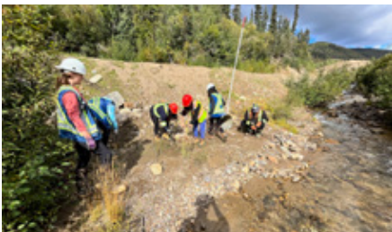
/ FNNND Participants planting willow stakes to control sedimentation and erosion on the banks of Dublin Gulch
