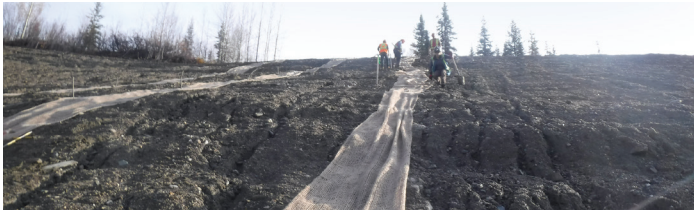
/ Control Pond jute fibre installation and seeding 2019
